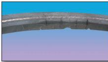
FIGURE 4: BELT UNDERSIDE CRACKED
