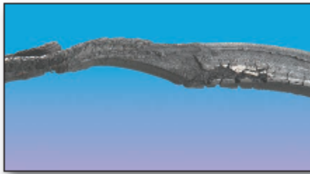
FIGURE 3: BELT SLIP BURN
